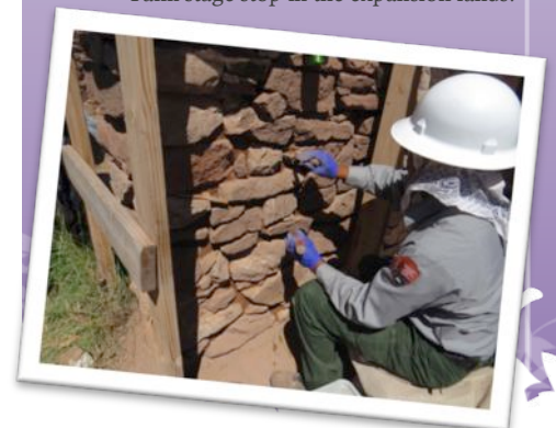
Masonry stabilization at the Depot Tank stage stop in the expansion lands.
